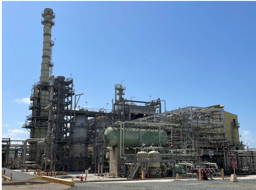
Low Sulphur Gasoline Plant
