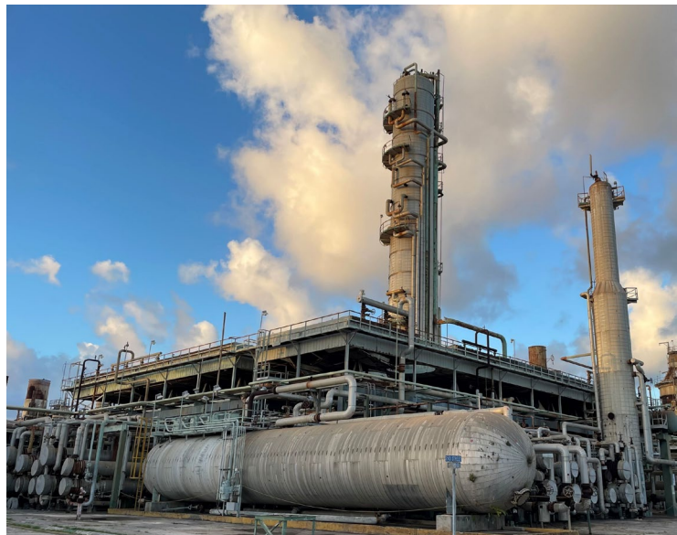
No. 2 Crude Distillation Unit
