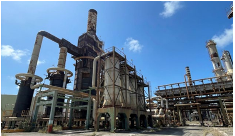
No. 2 Platformer Unit
